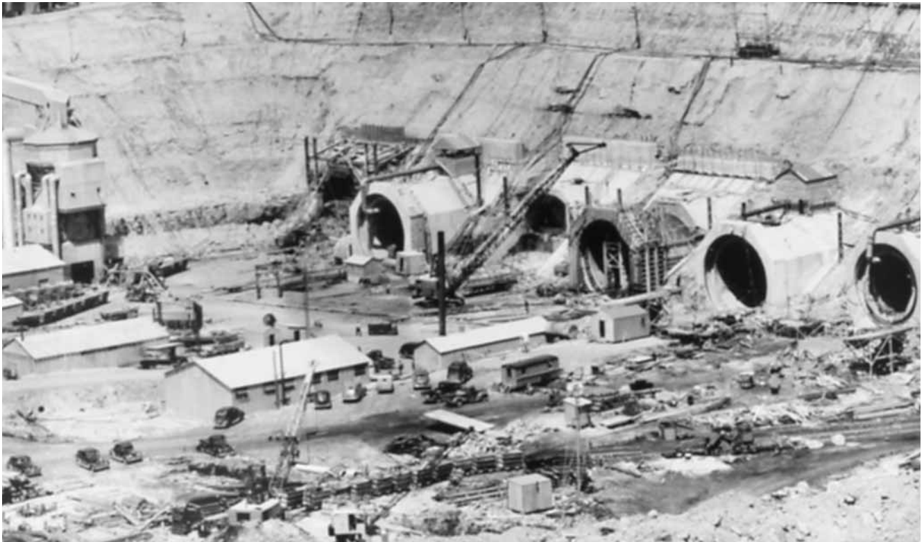
The Garrison Dam's massive, powerful tunnels under construction. Image courtesy of Marilyn Cross Hudson.
