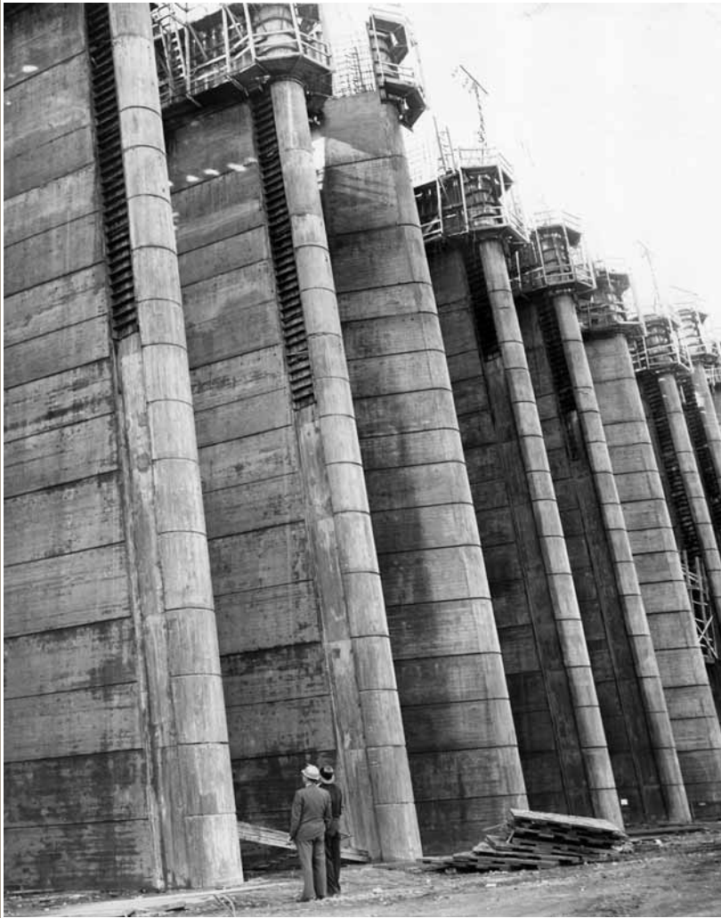
Water intake structures under construction at Garrison Dam, ca. 1950–1959. Image courtesy of Institute for Regional Studies, North Dakota State University, Fargo. Folio 69.09.05.
